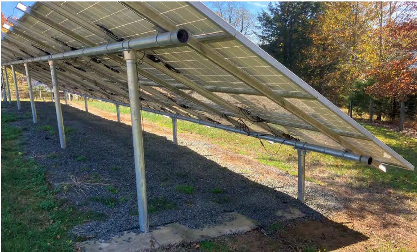
Concrete Foundation Beams and 3 Inch Pipe Structure
