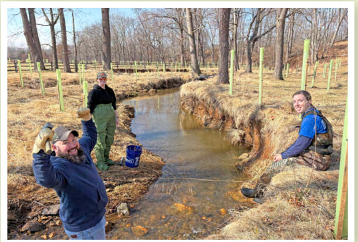
Volunteers waded into Bartons Creek during a "live staking" at Oakendale Farm, when tree cuttings are staked into the ground. Once grown, these trees will stabilize the heavily-eroded stream banks. Photo by Lea Justice
