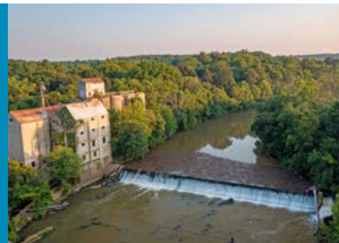
The Rapidan Mill on the Rapidan River in Orange County. While the current structure was built in the 1950s, the original mill on this site predated the Declaration of Independence. Photo by Hugh Kenny
