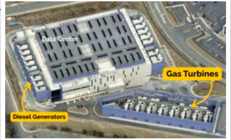
Vantage VA2 data center in Sterling, VA. Photo from Loudoun County online mapping tool
