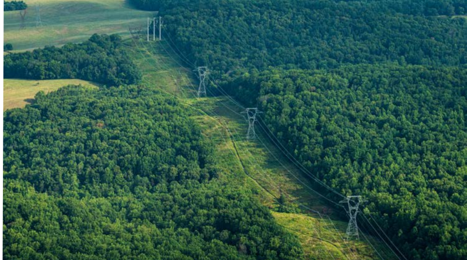
230 kV transmission line
