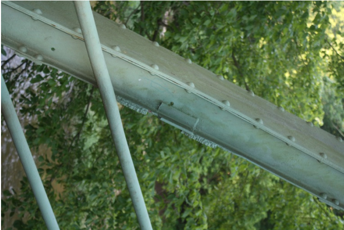
Existing welded plate repairs to end post.
