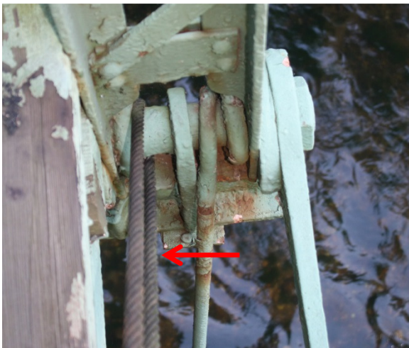
Detail of bottom chord connection with added cable and broken counter (denoted by red arrow).
