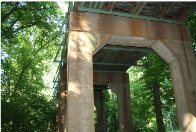
Overview of concrete bent.
