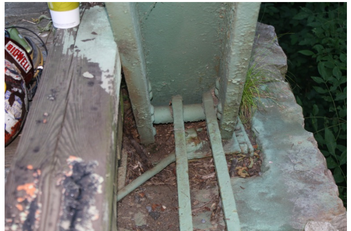
Expansion bearing (roller nest) and bottom chord connection at end post. Note minor buildup of debris.
