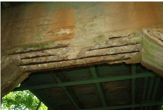
Typical example of spalling on a concrete bent.
