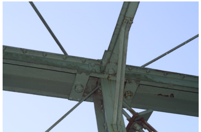
Top chord connection detail.
