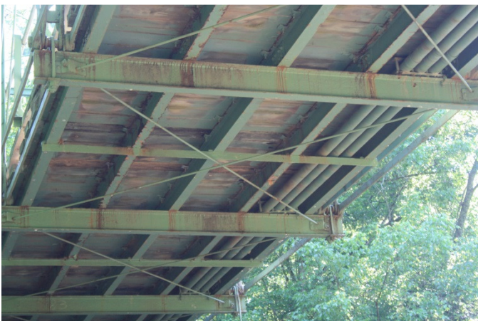
Overview of floor beams, deck stringers, and lateral bracing under the deck of the truss span.
