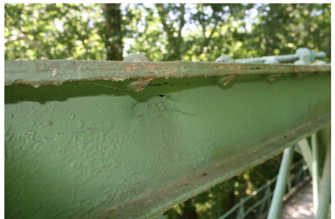
Isolated area of damage to top chord.
