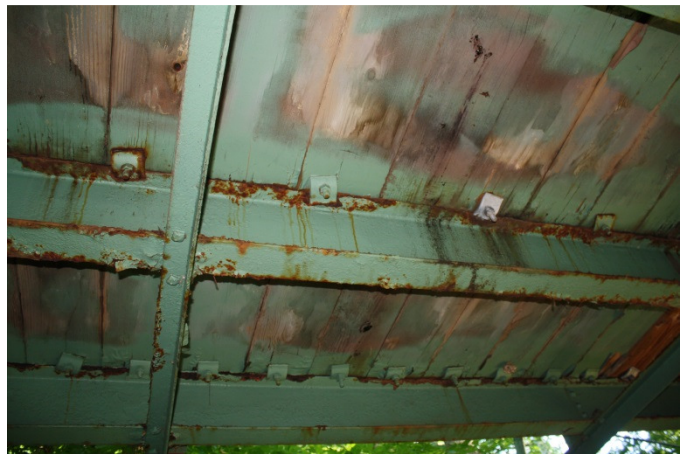
Detail of approach span stringer (typical).
