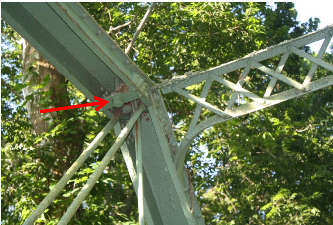
Top chord connection and portal bracing detail. Note pin for lateral bracing extending through the top chord batten plates (an unusual design feature of this bridge), denoted by red arrows. This detail is found at all panel points.
