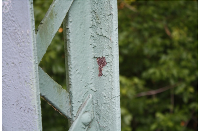
Vertical member detail showing rolled tee and riveted lacing. Note the use of angled ends on the lacing bars as opposed to rounded ends most commonly found on truss bridges.
