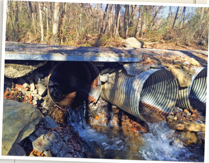
This is an example of a culvert that will be replaced by the brook trout restoration project because it prevents fish passage. Photo by Carolyn Sedgwick
