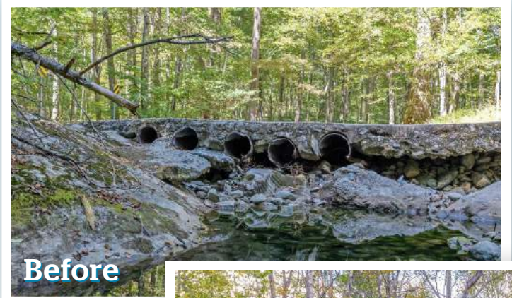
The old low-water concrete crossing and culverts before removal and the new open-span bridge after installation. Photos by Hugh Kenny
