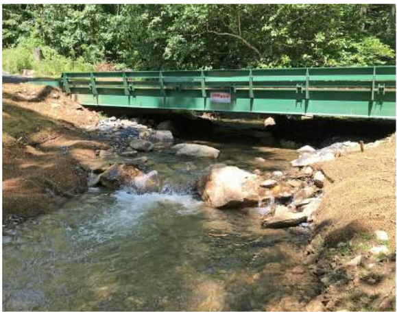
At Bolton Branch, this new bridge replaced an old concrete low-water ford. Photo by Claire Catlett
