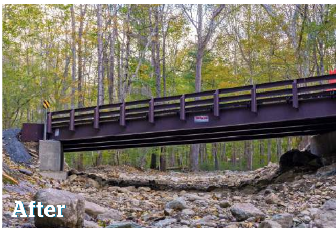
The old low-water concrete crossing and culverts before removal and the new open-span bridge after installation. Photos by Hugh Kenny
