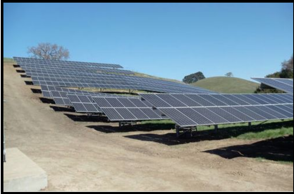
Figure 9: Ground-mounted solar arrays located on a hill, avoiding grading and fill.
