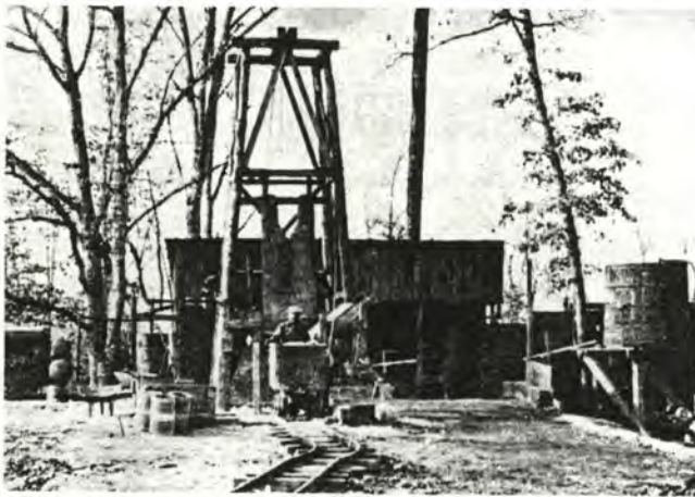
Figure 14. Surface plant during 1934 at the Melville mine, Orange County. (Photograph by C. H. Vivian, 1934, p. 4326)
