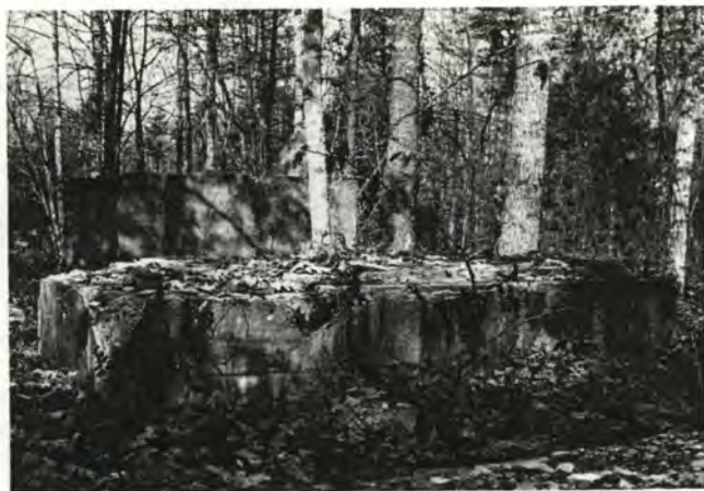
Figure 16. Concrete foundations at the old Wilderness mine, Orange County
