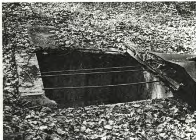
Figure 15. Water-filled, open shaft at the old Wilderness mine, Orange County
