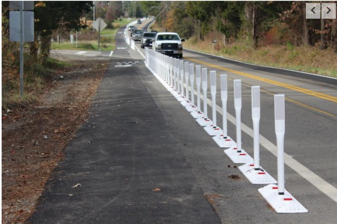
Bollards or delineators align Sinai Road separating a section of the road from traffic to allow for a pedestrian walking area. The speed limit also has been reduced to 35 miles per hour on the same stretch of road.
