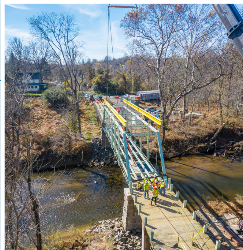
Contractors fly the restored metal truss Waterloo Bridge back onto its stone abutments. Photo by Hugh Kenny
