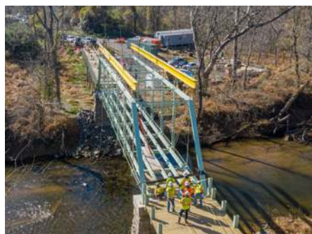
CONTRACTORS FLY THE RESTORED METAL TRUSS WATERLOO BRIDGE BACK ONTO ITS STONE ABUTMENTS. Photo by Hugh Kenny
