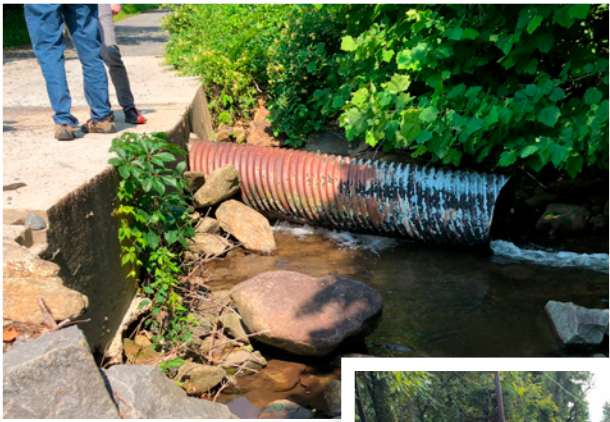
▲ BEFORE: Stream flow and fish passage is restricted to one undersized culvert. Photo by Claire Catlett.
