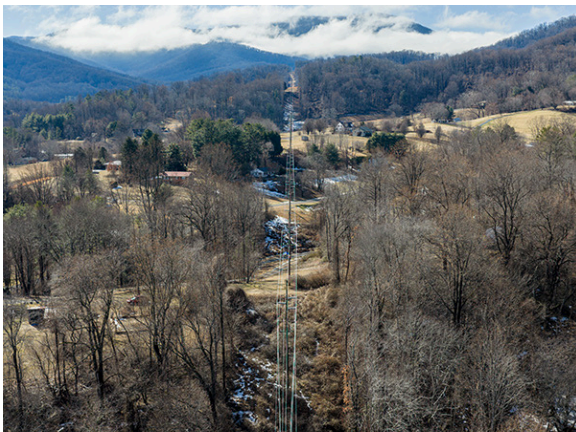
Existing transmission line in Sperryville. Photo by Hugh Kenny, PEC.
