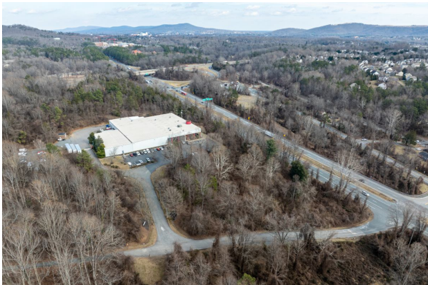
Albemarle County has identified potential Data Center Overlay Districts, including near the I-64/US29 interchange. Credit: Hugh Kenny, PEC.
